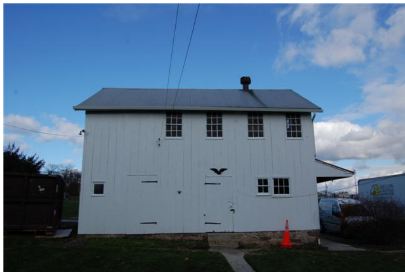
Rear building with no fire damage Photo # 11
