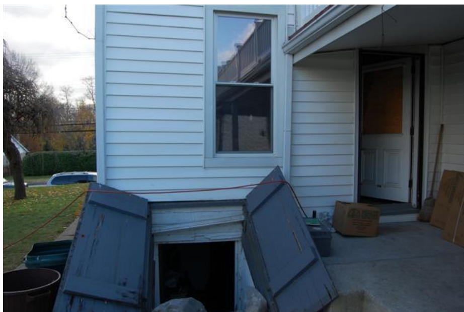
Basement entry and rear door to house Photo # 16
