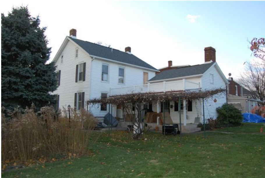
Rear and east side of house Photo # 13
