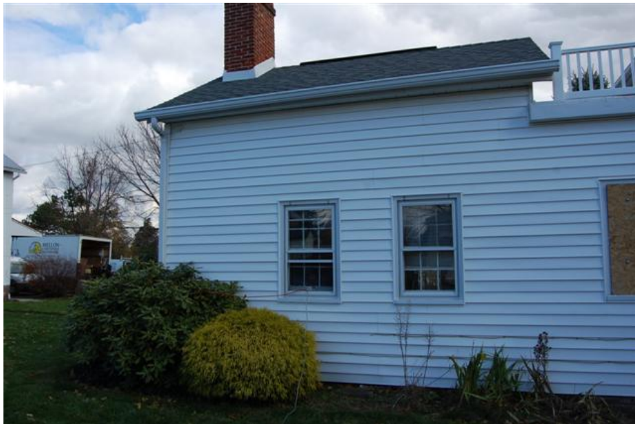
West side rear of house Photo # 5
