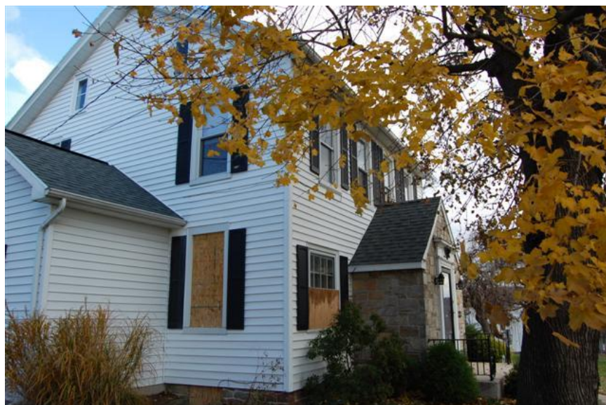
West side exterior view of house Photo # 3
