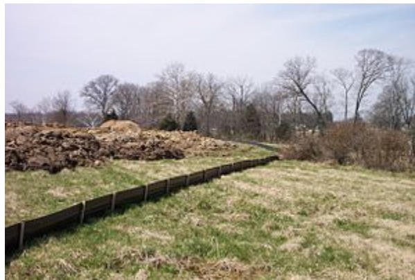
Construction Runoff Fence via Wikipedia
