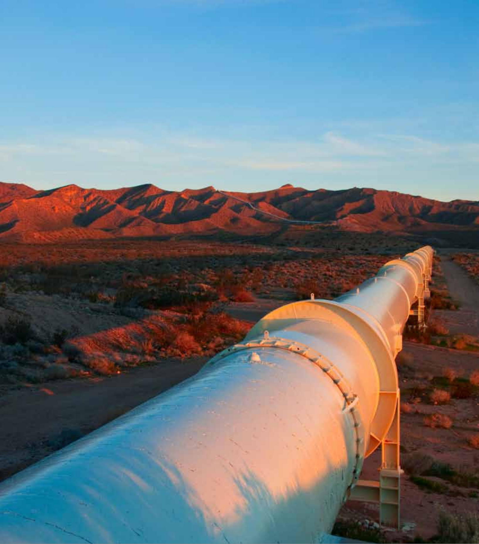
COVER IMAGE: The Keystone Pipeline System is a pipeline system to transport synthetic crude oil and diluted bitumen ("dilbit") from the Athabasca oil sands region in northeastern Alberta, Canada to multiple destinations in the United States, which include refineries in Illinois, the Cushing oil distribution hub in Oklahoma, and proposed connections to refineries along the Gulf Coast of Texas.
