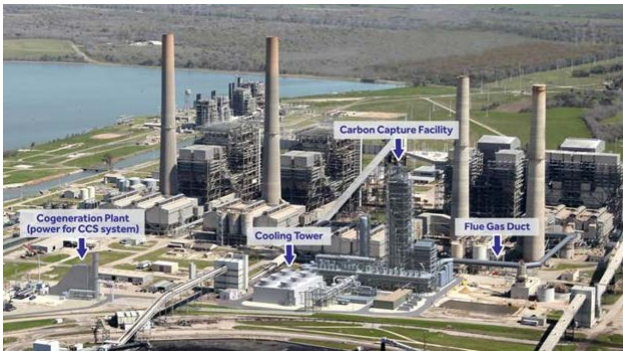
Figure 18: Petra Nova CO 2 Capture and Sequestration Project Layout
